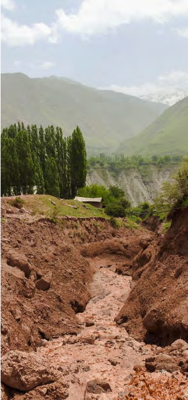
A small headwater stream of Vakhsh River brings heavy loads of sediment into the river system after receiving a spring rainfall. This sedimentation is reducing the capacity of Tajikistan's Nurek reservoir, and threatening the long term viability of a nationally important hydropower operation.
