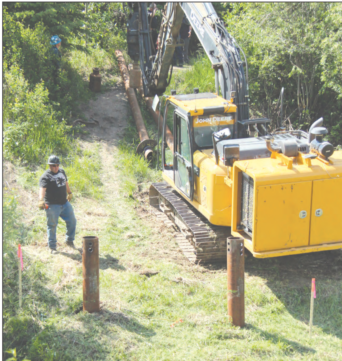
Crews drive pylons for a new footbridge on the north bank of Dawson Creek.
