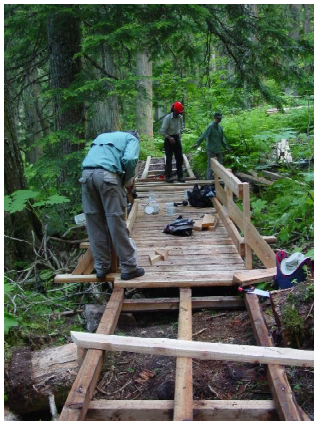
Laying down the first boards in July, 2010.
