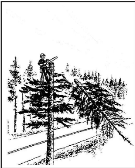
Removing the hazardous portion of a tree along a road. Tree can be “jagged-topped” with a chainsaw.
