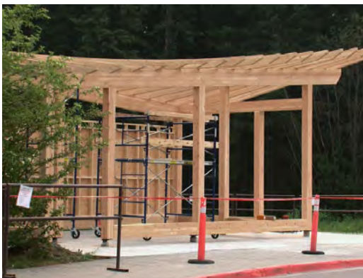
Figure 2.9 UNBC Bus Shelter Under Construction
